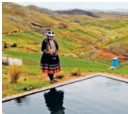
Water harvesting. During the rainy season, useless runoff water is stored in ponds.
